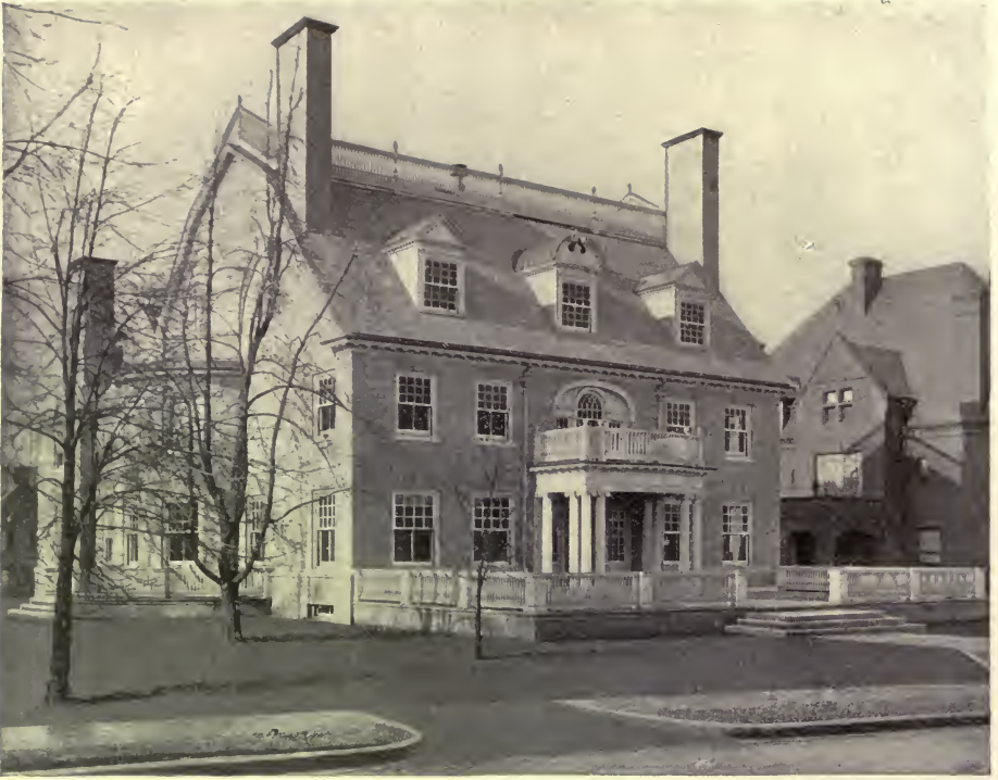
FIG. 26.—HOUSE IN PITTSBURG.
