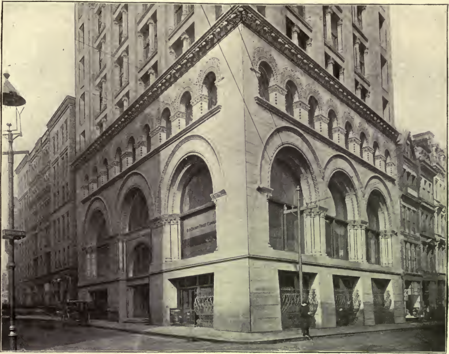
FIG. 24.—LOWER PART OF AMES BUILDING,
