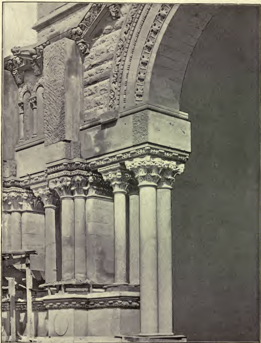
FIG. 49.—DETAIL OF PORCH—TRINITY CHURCH.
