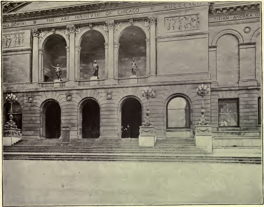
FIG. 28.—MAIN ENTRANCE TO ART INSTITUTE.
