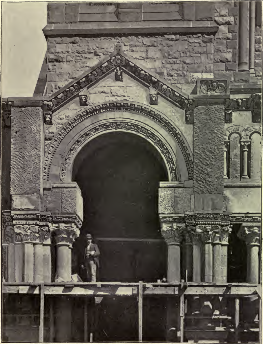
FIG. 47.—NORTHWEST ARCH OF PORCH, TRINITY CHURCH.
